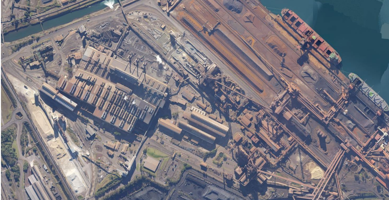
Figure 2.1 – Aerial photograph of the Ironmaking department of BSL Steelworks
