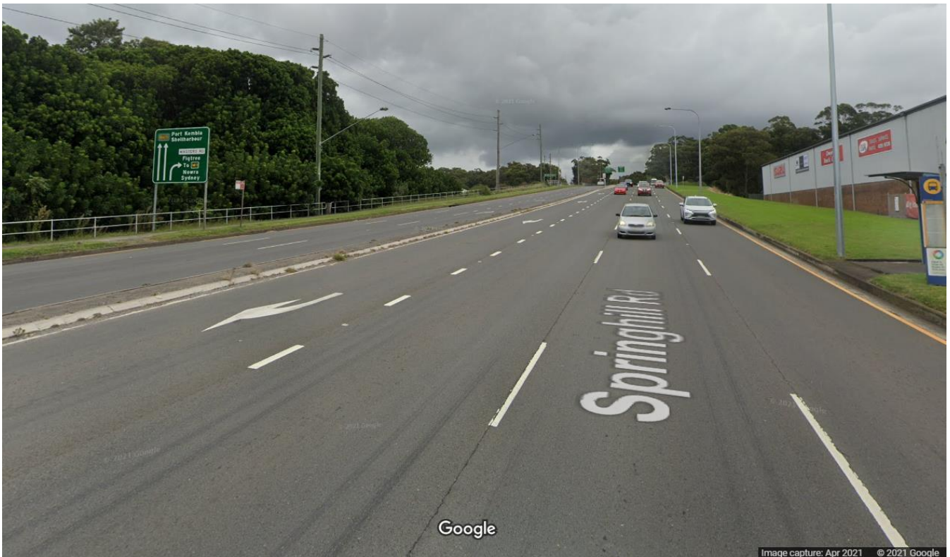
Figure 4.5 Springhill Road, viewed westwards from BlueScope North Gate
