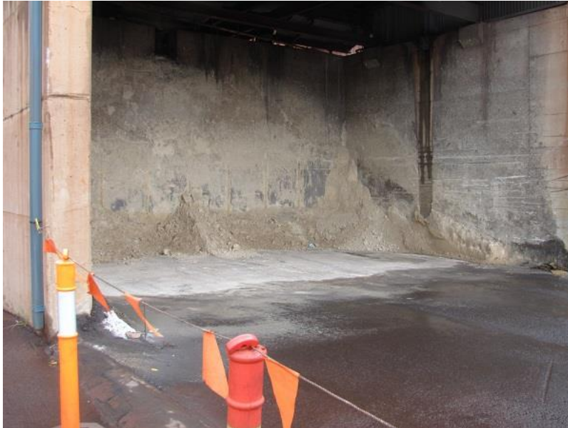
Photograph 5 Storage Area for Gypsum (24 February 2022)
