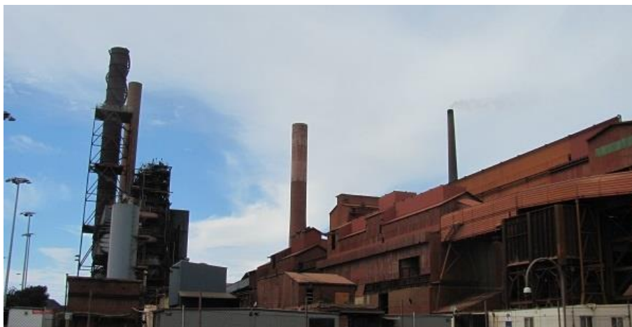
Photograph 2 Sinter Plant and WGCP (1 March 2019)
