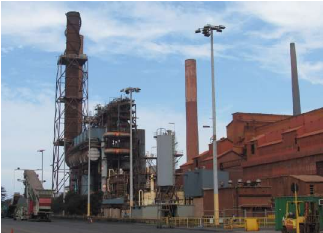
Photograph 2 Sinter Plant and WGCP (10 March 2016)
